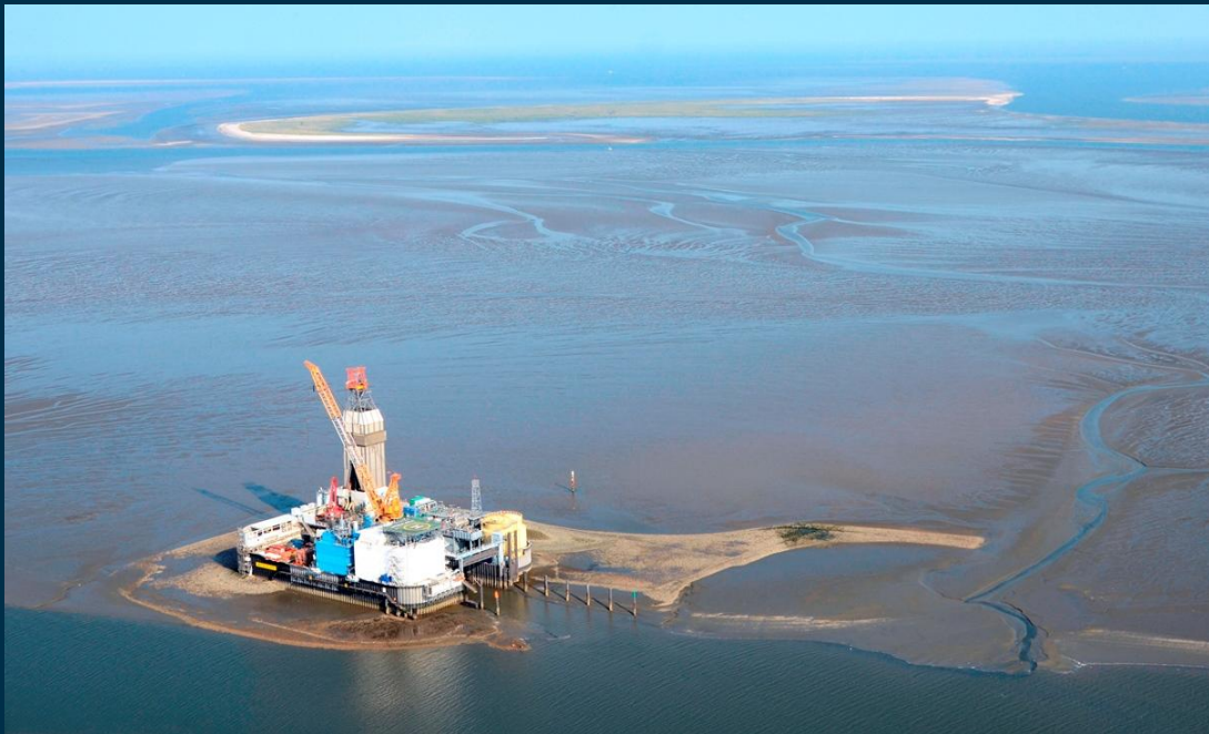
Photo: Media library www.Mittelplate.de . Oil platform Mittelplate.
