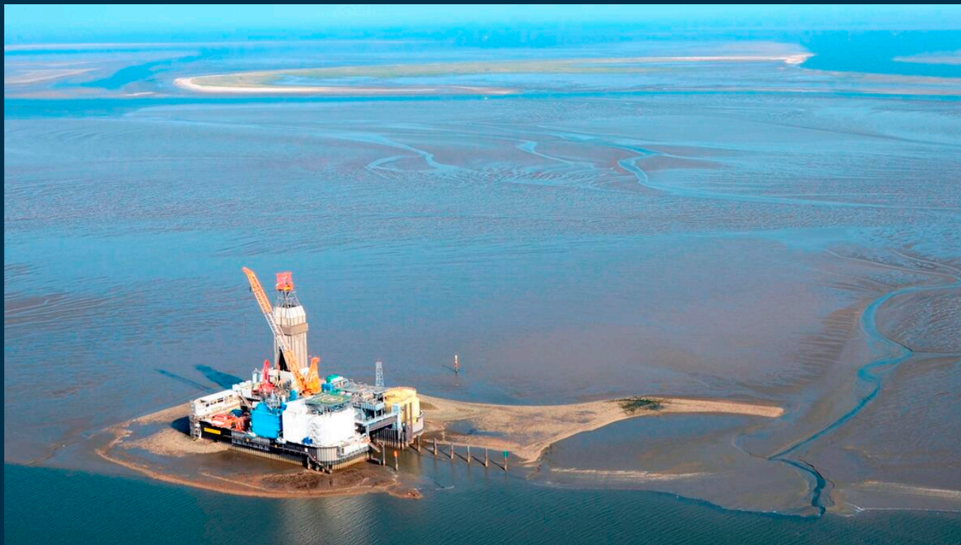
Photo: Media library www.Mittelplate.de . Oil platform Mittelplate.
