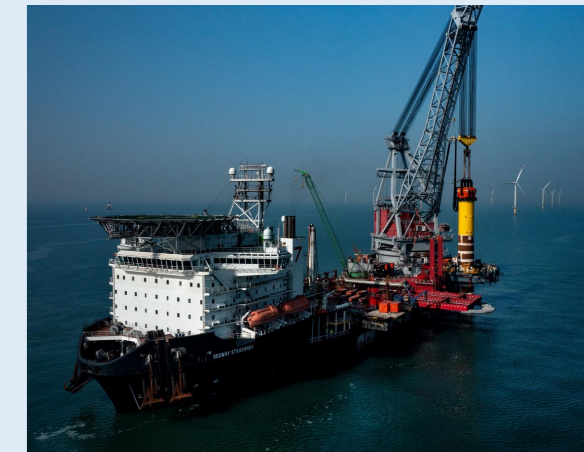
Fig. 3 Installation ship during offshore wind park construction. (Source: RWE)
